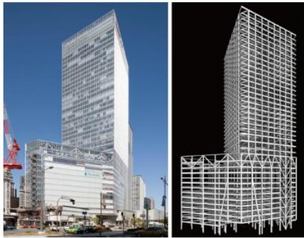
Figure 11. Tokyo BRBF (Gran Tokyo North).
