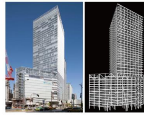
Figure 11. Tokyo BRBF (Gran Tokyo North).
