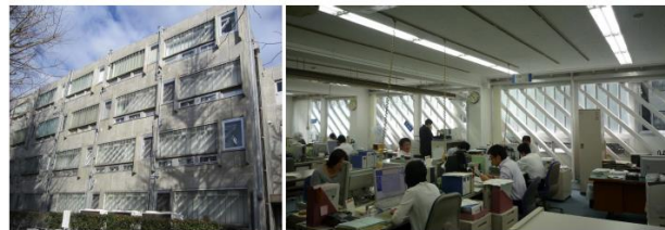
(a) Exterior appearance
