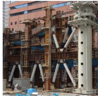
Figure 12. Erection of large BRBF.
