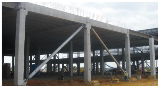
Typical buckling-restrained braced frame.
